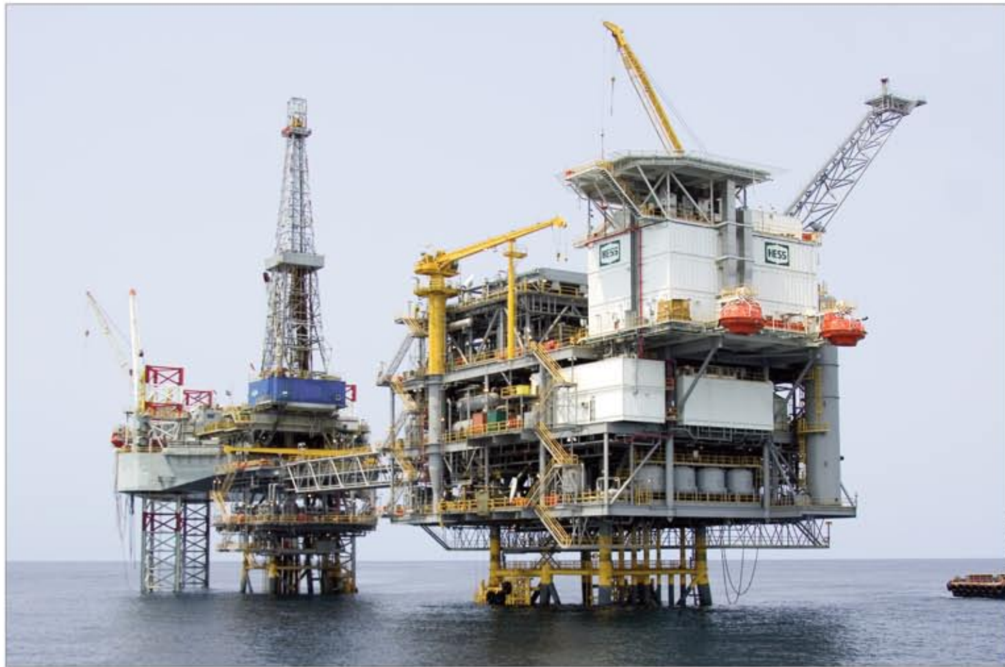
The Okume Complex Development is a large-scale industry program with three fixed platforms, two tension leg platforms and a central processing facility. Through this development, Hess has demonstrated a long-term commitment to building a strong local staff and contributing to the community in Equatorial Guinea.
